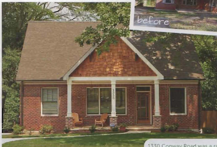
1330 Conway Road was a ranch to bungalow whole-house conversion. Epic Development removed the roof, raised the ceiling heights on the first floor from 8 to 9 feet, and added two bedrooms and baths.
